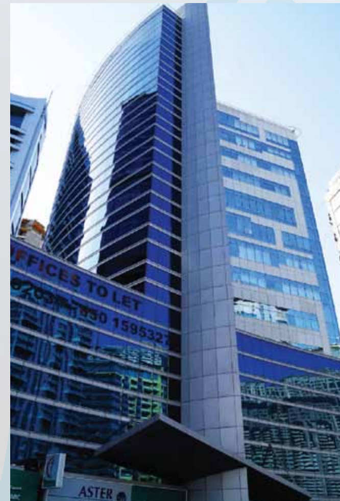
COMMERCIAL / OFFICE BUILDING 2B+G+3P+11-ICON TOWER, TECOM, DUBAI
